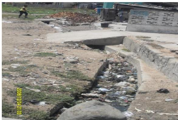
**Plate 6: A choked gutter**
